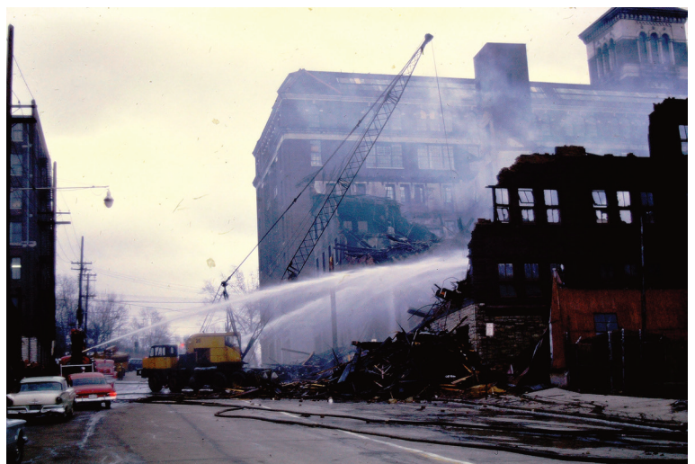
The remains of the Baldwin fire on the morning of March 5, 1964. Photo Cincinnati Enquirer.
